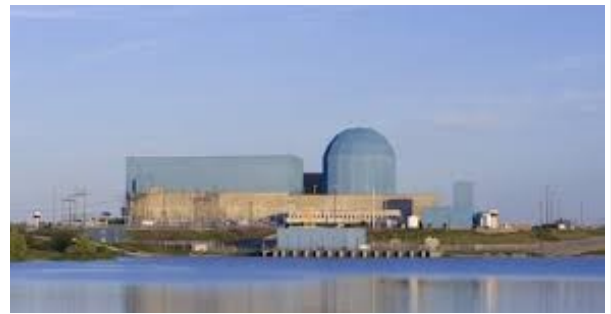
Clinton nuclear plant
